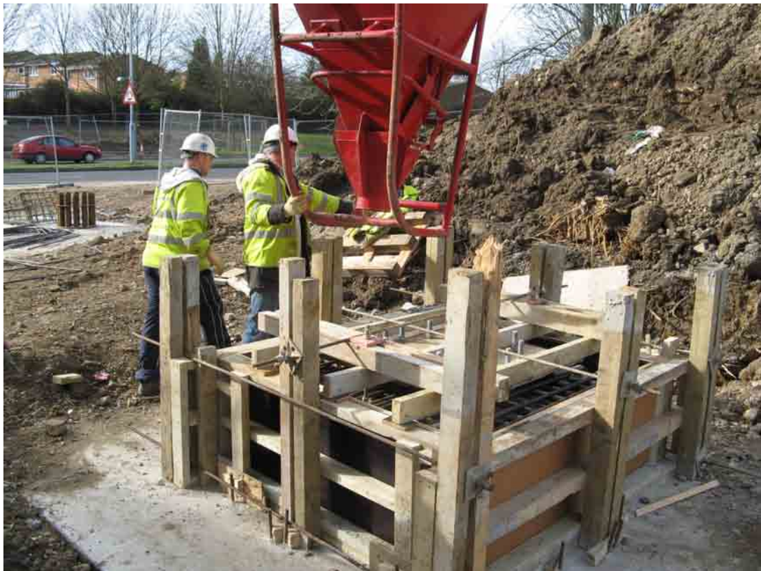
Photo 2: Using a hopper to place concrete to a column plinth
