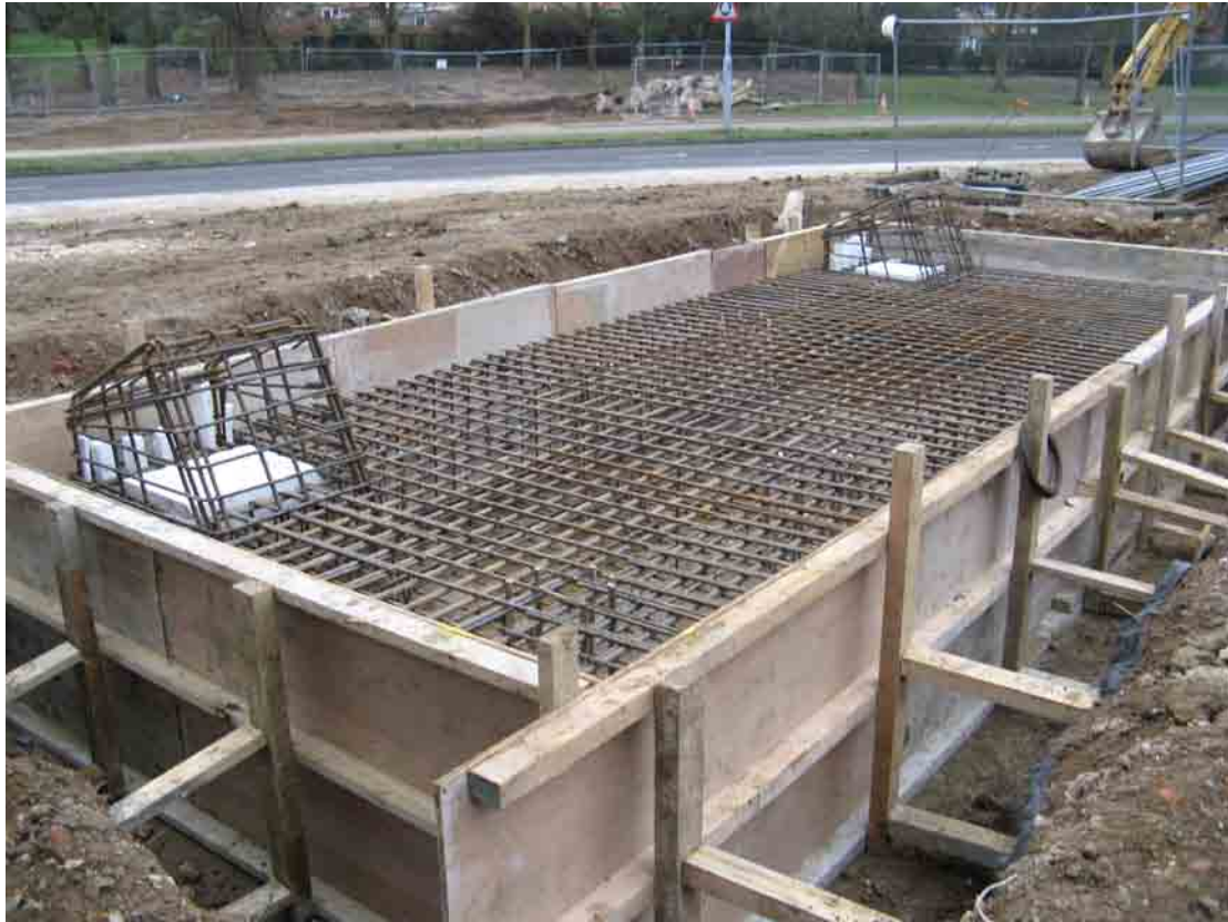
Photo 1: Steel reinforcement in place for the main arch base
